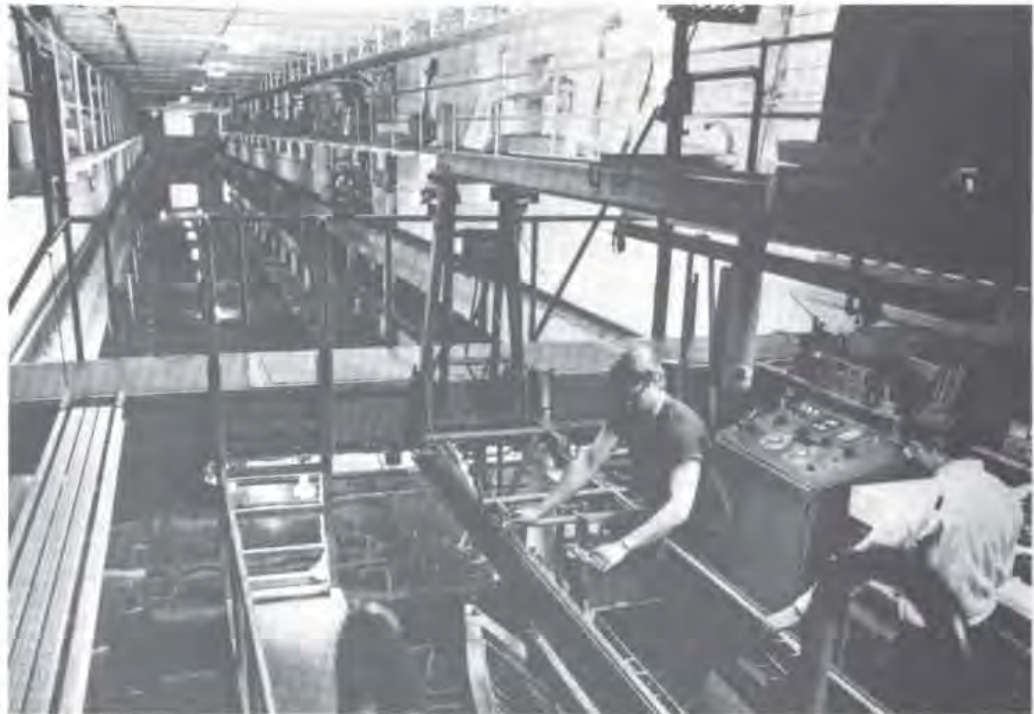
FIGURE 1.12. Marine engineers testing ship hull designs in a towing tank. (Courtesy University of Michigan College of Engineering)
